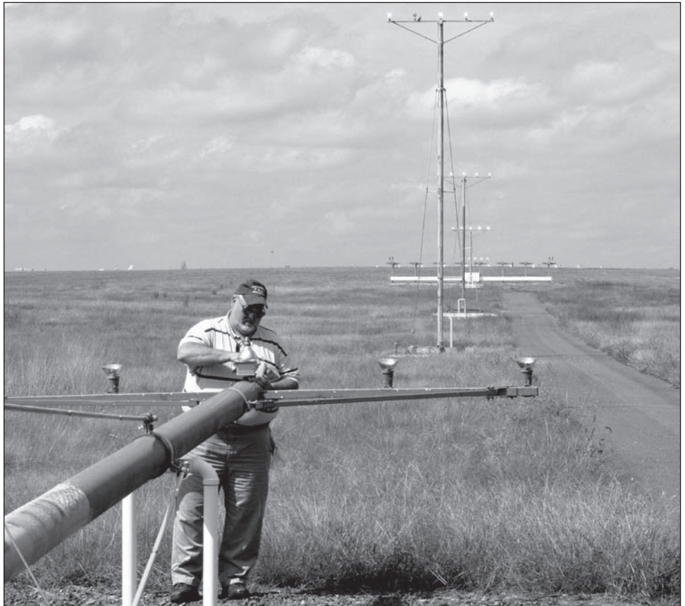
Figure 1: A Technician Conducting an Equipment Check
