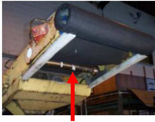
Figure 2 - Roller located under the conveyor belt
